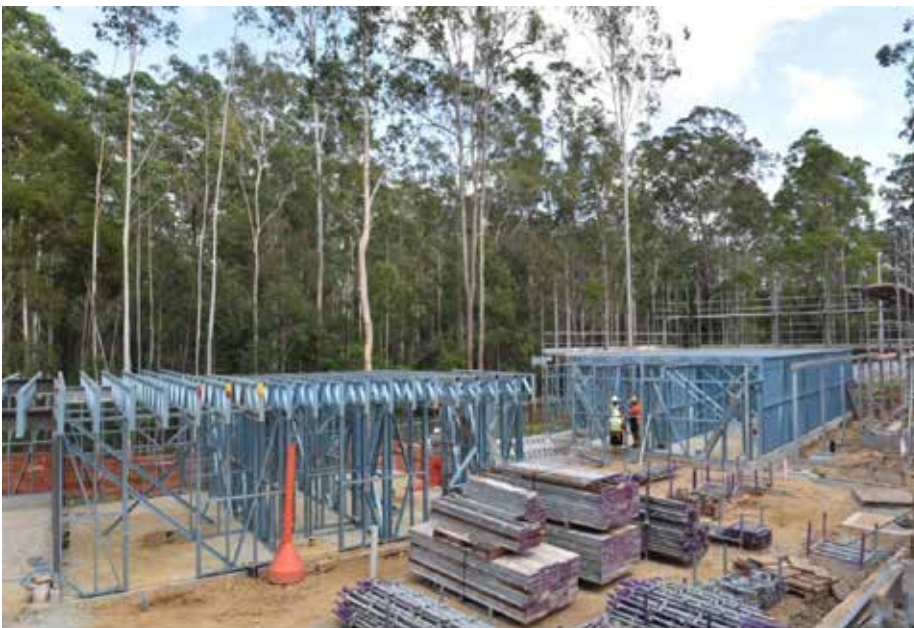
Concrete slabs poured and wall, floor and ceiling frames are set.
