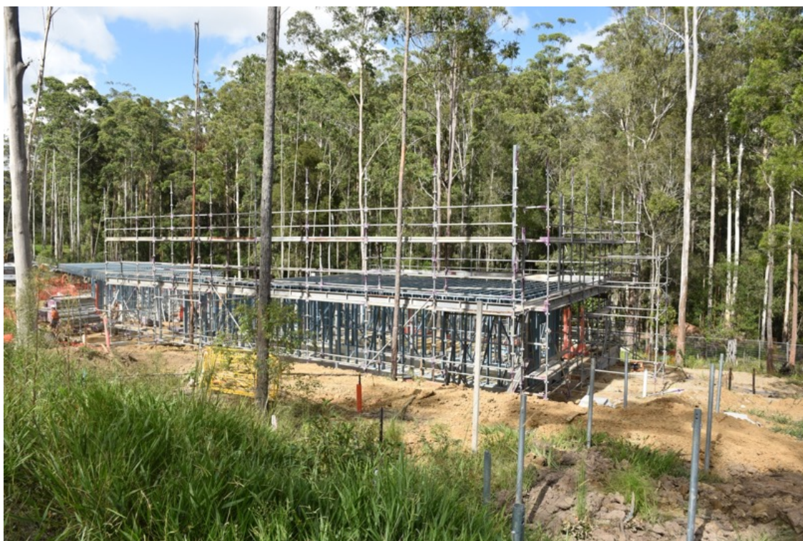
North building of the complex under construction.
